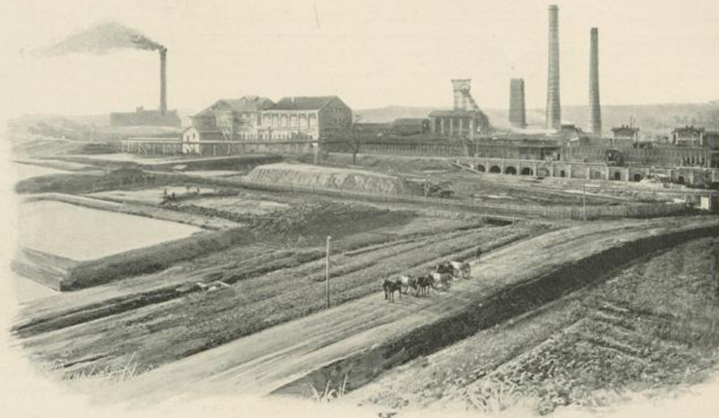
Ignaz-Schacht in Ellgoth.
