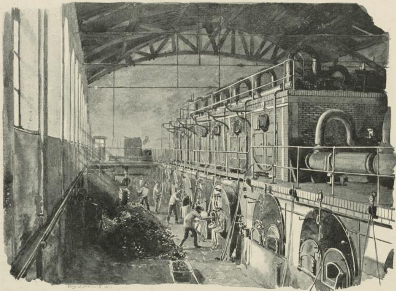
Kesselhaus in Iserthal
